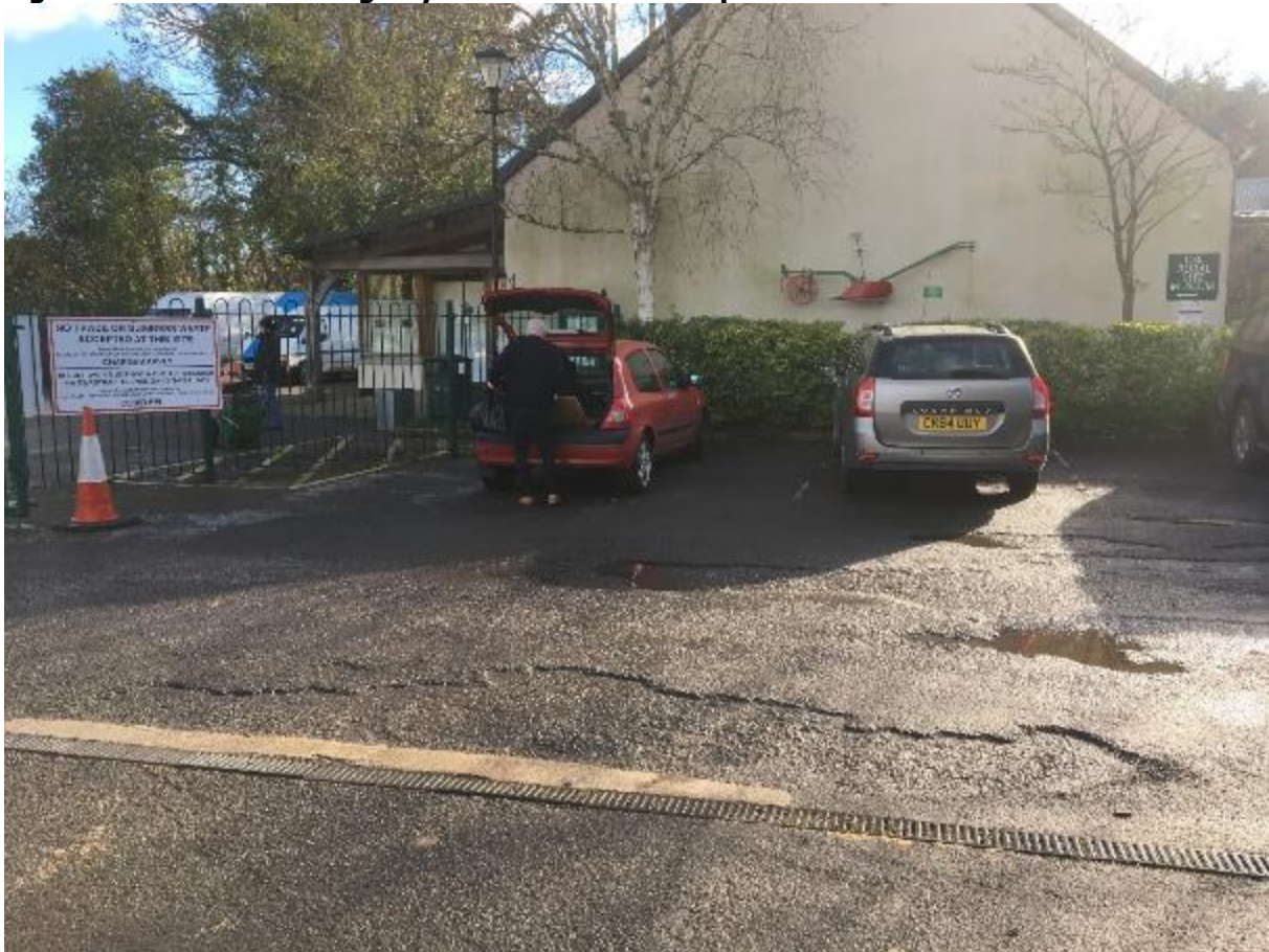
Figure 31: Marked Parking Bays in the Additional Operational Area
