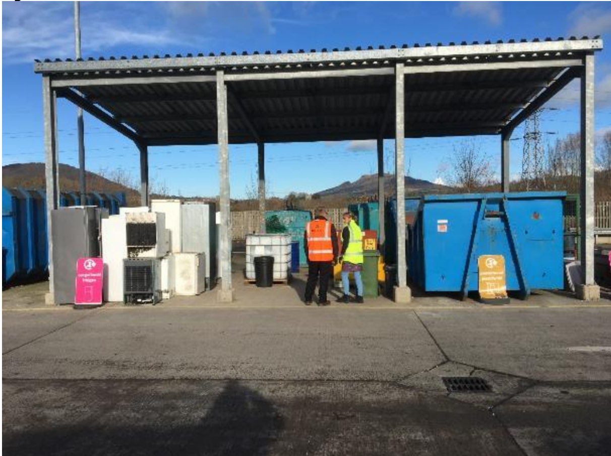
Figure 19: Central Covered Area
