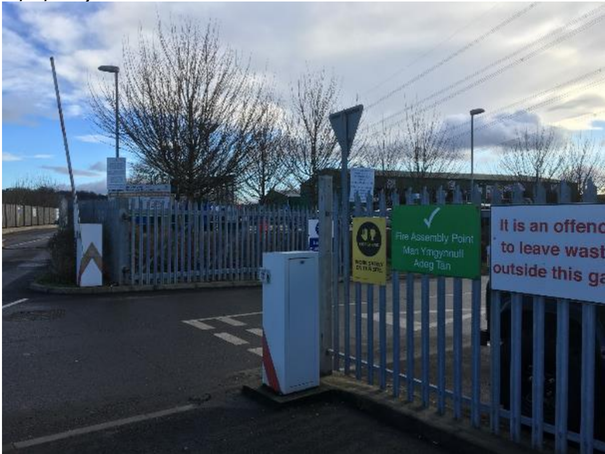
Figure 12: Separate Llanfoist WTS and HWRC Service Entrance / Exit (E.How 31/02/2019)
